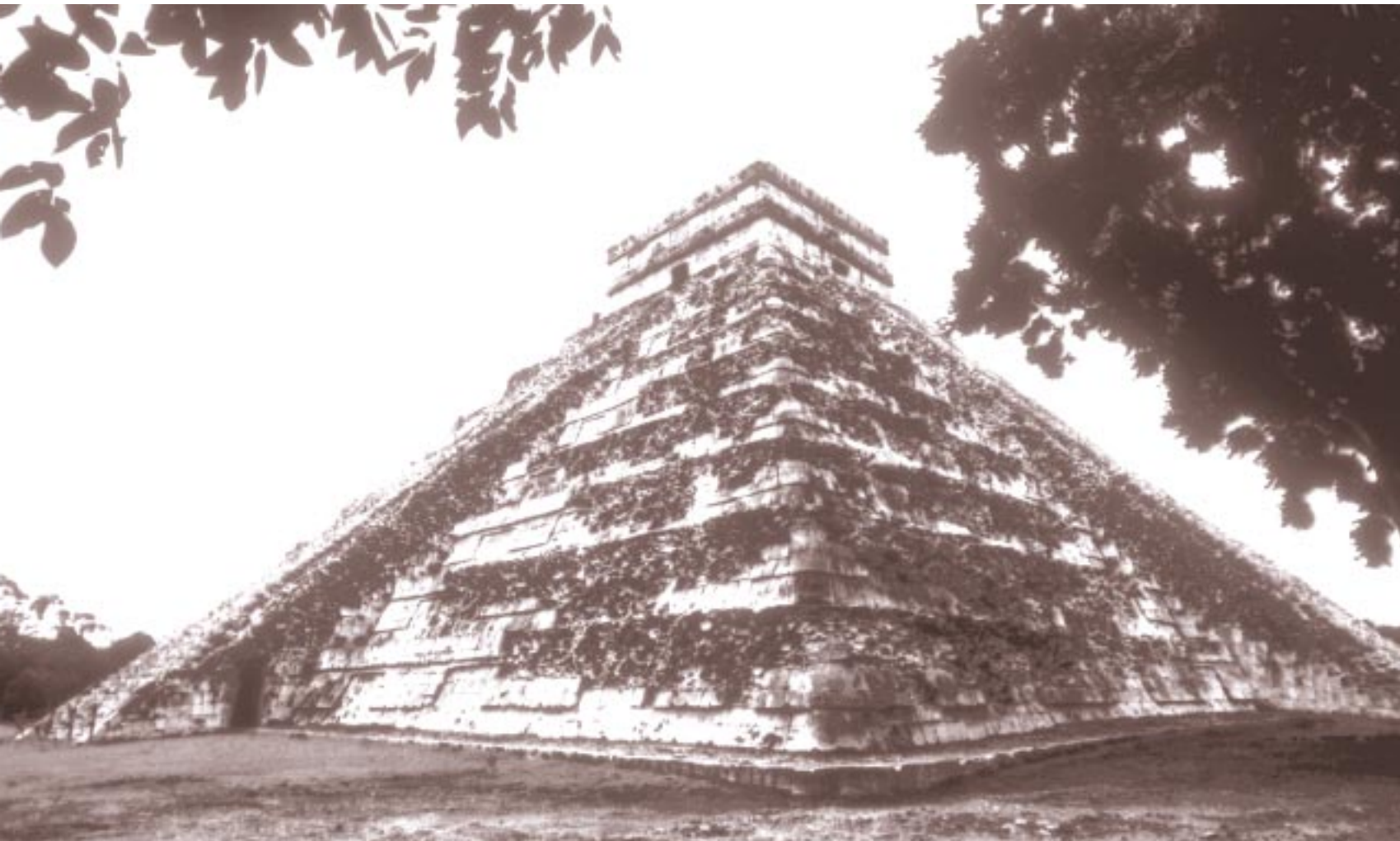
A component of the restoration program of Kukulcán's pyramid—begun in the mid-1920s—was the removal of the trees and shrubs that had taken root in the nooks and crannies of the stonework.
