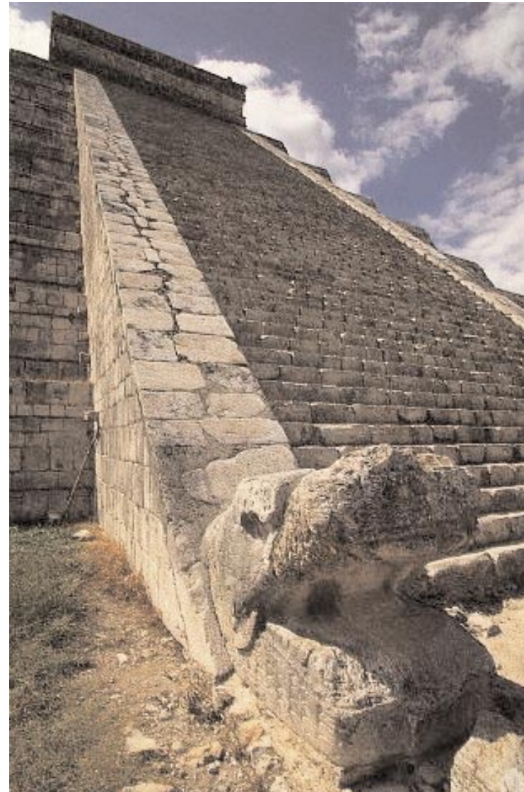
The faces of the individual steps of Kukulcán are sloped at an angle of approximately 73 degrees. Note the serpent’s head at the base of the stairs.
