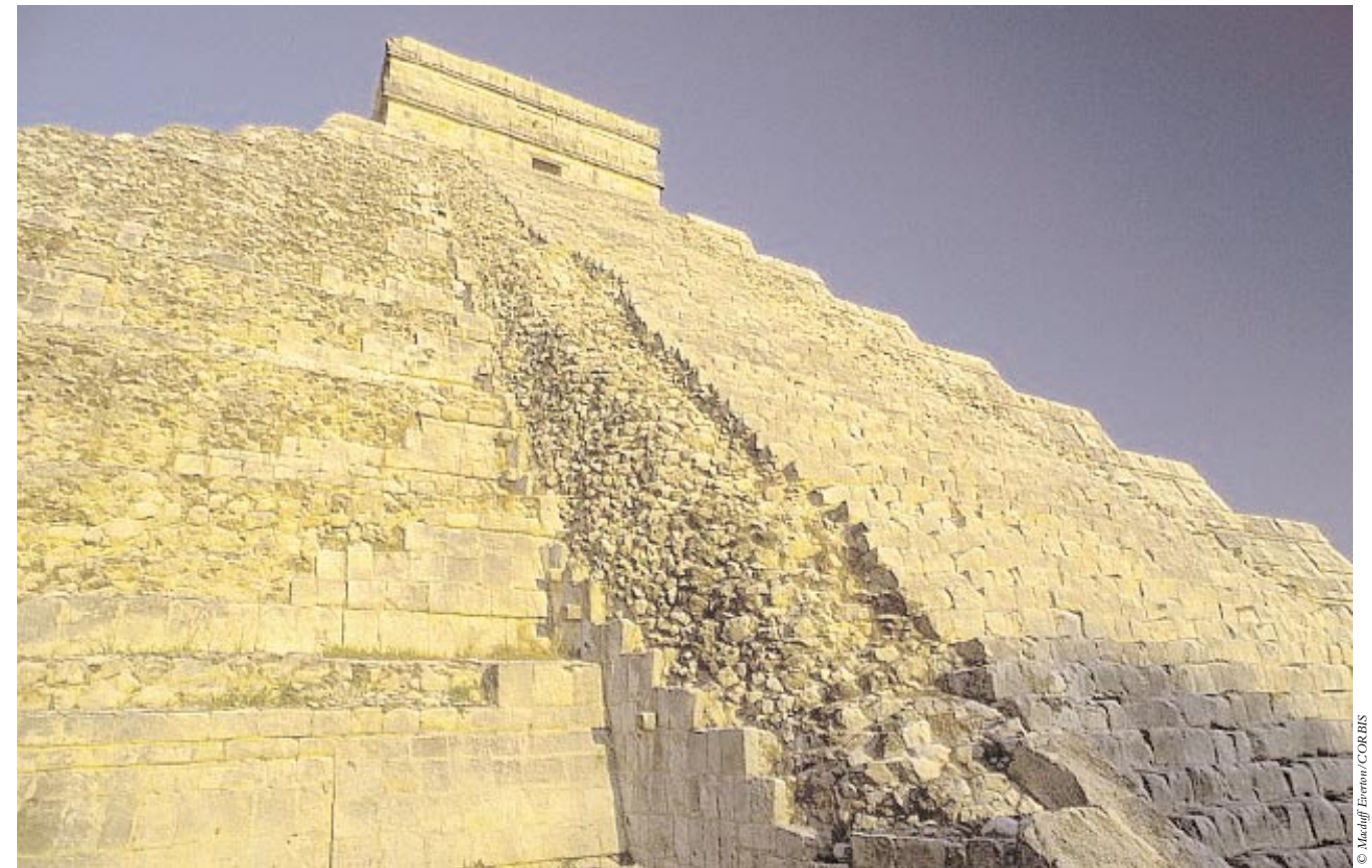
Behind the exterior casing stones the construction of Kukulcán appears to consist of stones of an irregular shape that were not carefully cut or fitted, the crevices and interstitial spaces filled with rubble and lime mortar.
